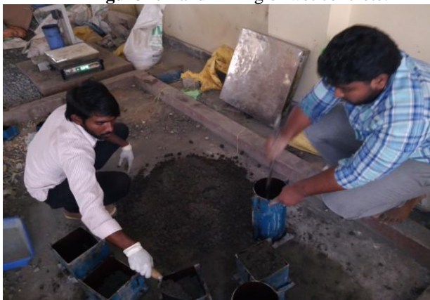
Figure 2. Placing of wet concrete in moulds.
