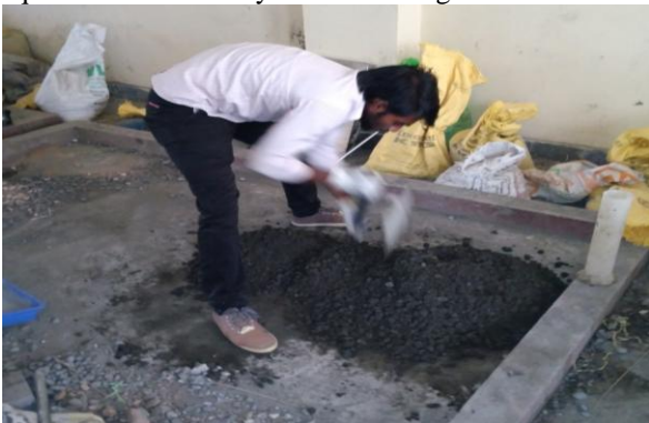
Figure 1. Hand mixing of wet concrete.
