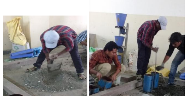
Fig 3.2: Hand mixing and placing of concrete mix
